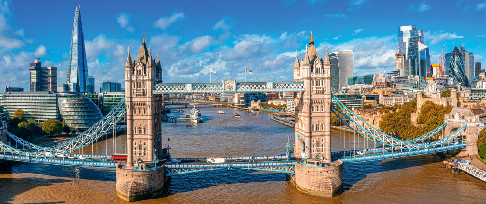
London, Tower Bridge © ingusk - stock.adobe.com
